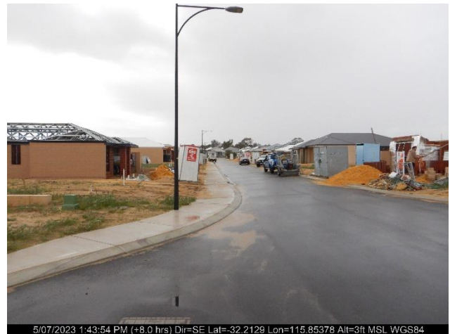
Photo ID: Photo 2 Looking across the subdivision site with lots where construction on new builds has commenced.
