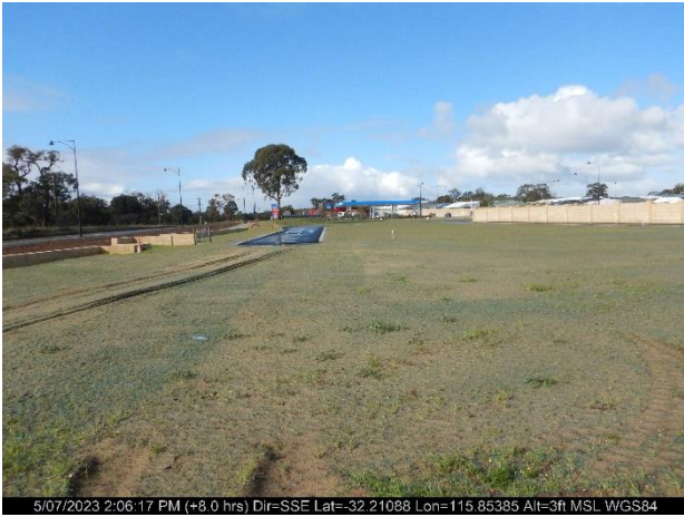
5/07/2023 2:06:17 PM (+8.0 hrs) Dir=SSE Lat=-32.21088 Lon=115.85385 Alt=3ft MSL WGS84 Photo ID: Photo 5 Looking across the land north-east of the lot which is cleared and ready for new dwellings.
