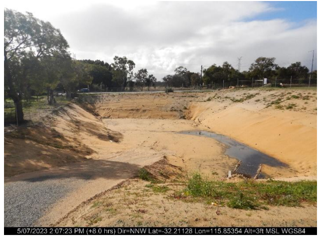
5/07/2023 2:07:23 PM (+8.0 hrs) Dir=NNW Lat=-32.21128 Lon=115.85354 Alt=3ft MSL WGS84 Photo ID: Photo 6 Looking at the drainage sump.
